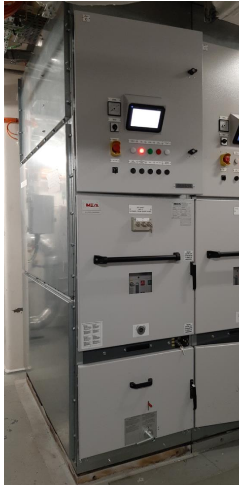
Figure 60: Additional circuit breaker (ACB “B”) installed in the MSB room
