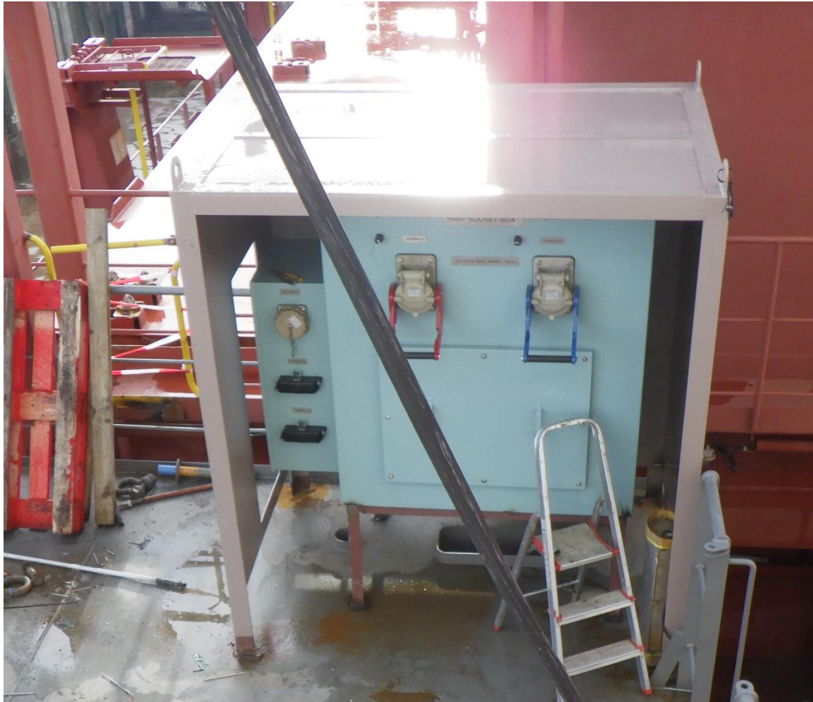
Figure 48: AMP socket box onboard a vessel, containing only the receiving socket for the connection of the cable from ashore
